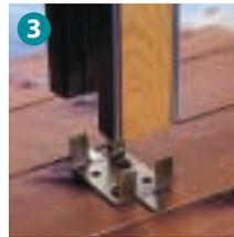
**Self-adjusting floor plates** Long vertical fingers slide into the studs allowing for floor settlement without disturbing the horizontal alignment of the header and track.
