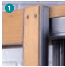
**Steel-wrapped studs**, nailed to the pre-assembled header, give maximum rigidity and restrict accidental nail penetration.
