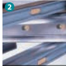
**Keyhole slots** in the aluminium box-section track allow easy removal (without damage to the wall) in the unlikely event of this being necessary.
